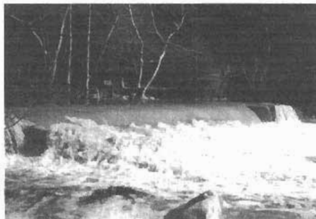
Niles Dam—Alameda Creek
