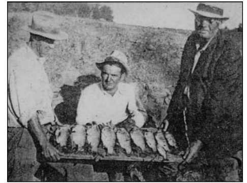
Workmen building Calaveras Dam in the 1920s pose with steelhead caught during a lunch break. Photo courtesy SFPUC.
