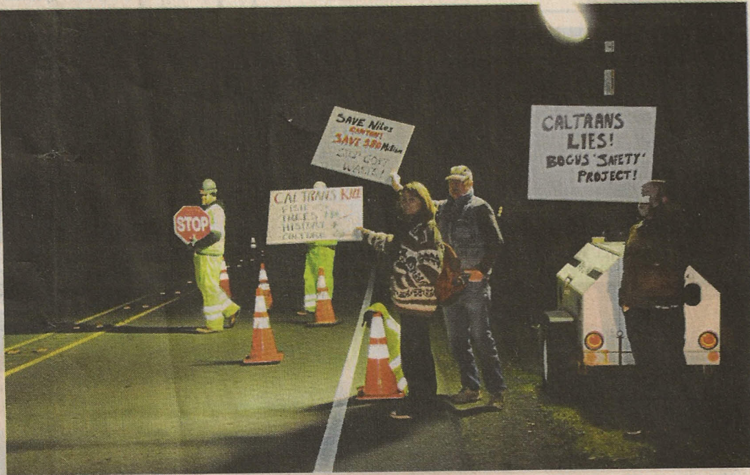
Protestors were on hand to picket crews cutting down trees along Niles Canyon Road.
