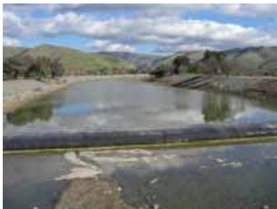
Inflatable dam in Alameda County flood control channel. Photo by Brian Sak.
