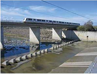
*"Dragon's teeth" under the BART weir. These concrete blocks break up high flows and slow velocities in the flood control channel. Photo by Brian Sak.*
