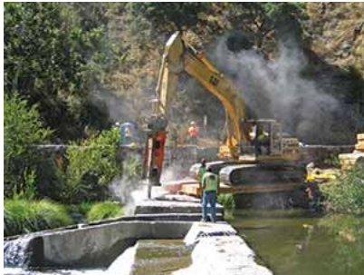
In 2006 the San Francisco PUC removed Sunol and Niles (pictured) dams from Alameda Creek, alleviating public safety concerns and providing steelhead and other fishes' access to upstream waters. Photo: Brian Sak.
