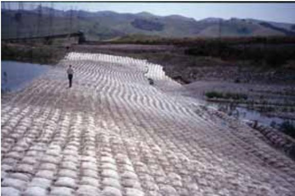
PG&E is moving forward with a project to remove a concrete mat at a pipeline crossing of Alameda Creek in the Sunol Valley. PG&E is coordinating the project with the SFPUC, which recently published a restoration report for the Sunol Valley, and with the Sunol gravel quarry operator, which will install cutoff walls along the quarry pits adjacent to Alameda Creek to prevent
