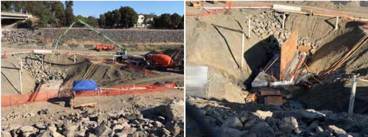
The first of three years of construction is well underway on the major fish ladder project in lower Alameda Creek. This fishway will allow steelhead and salmon to bypass the 12' high BART weir and the adjacent rubber dam. Contractors for ACWD are currently excavating and pouring foundations to anchor the lower end (the entrance) to the eventual fish ladder.
