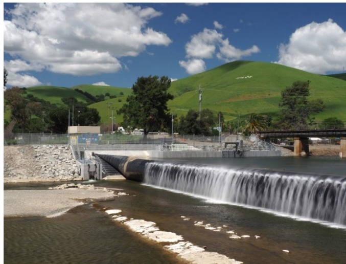
Figure 1 RD3 4/9/2019. Under normal operations, RD3 inflated with ~ 70 cfs overtopping flow. Ladder operational in the background
